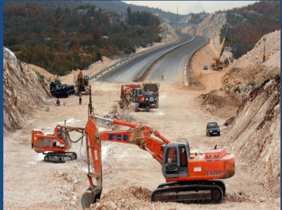
Construction of the Bar - Boljare highway
